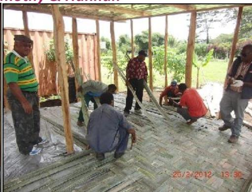
*Photos of various stages of the construction of the Temporary Dormitories made from bush materials (with bamboo flooring, right)*
